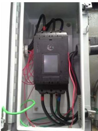
A synergy unit was installed on their Blanchard #2 grinder as an initial test with the target of saving 5% of the energy. A SGY-203 was installed on the 75HP motor, the installation was fast and easy utilising the 2.5" touch screen and automatic set up. Initial
